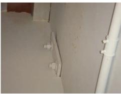
The mezzanine floor sheathing is separated from the concrete building wall up to 3/4"
