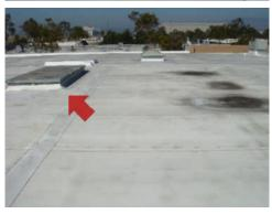
**PHOTO # 4** The roof deck has low areas causing puddling.
