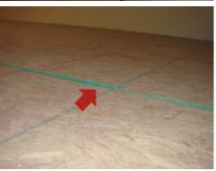
The framing below could be the cause of the uneven floor sheathing.
