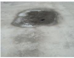
PHOTO # 8 [FE] Puddling noted at the front of the building unit at the left and right areas.
