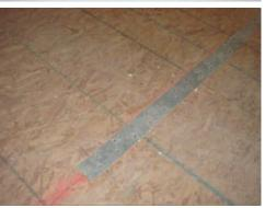
[FE] Void /gap at the front left corner of the mezzanine OSB sheathing.
